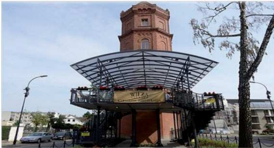
FIG. 3. Restaurant and café located in the water tower
